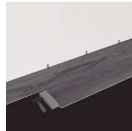
Step 8c: The product is properly locked when the two boards are flush across the top. Finish installing this plank tapping it with a tapping block on the long side to ensure secure installation.
